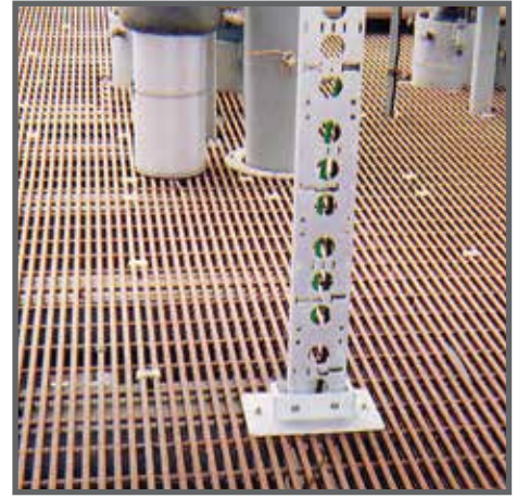
Offshore Oil & Gas Platform
